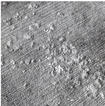
**Scaling** is caused when water freezes in the pores and capillaries in concrete. When the hydraulic pressure of the expanding ice exceeds the tensile strength of the concrete, scales of mortar detach from the surface, exposing aggregate.
