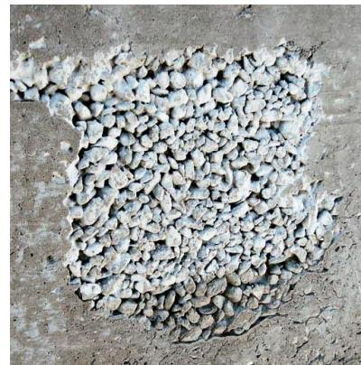
A **honeycomb** is a cluster of coarse aggregates where mortar did not penetrate. The aggregates are tightly packed but unbound, with poor compressive strength and negligible tensile strength. The aggregates need to be removed with power tools down to bare concrete, then filled.
