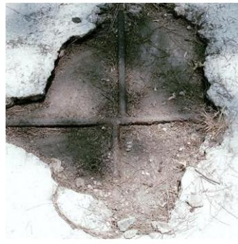
**Spalling** is similar to scaling, except the expansion occurs from deeper within the concrete, causing the surface to disintegrate into larger fragments. Common causes are rebar corrosion due to carbonation, intense heat that causes water vapor to expand violently, improperly constructed joints, and crack deterioration.
